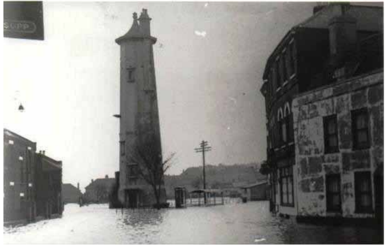
Flooding around the High Lighthouse (1953) © The Harwich Society
